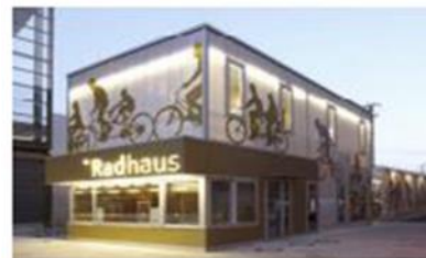
(iii) Radhaus building in Erfurt, Germany.
