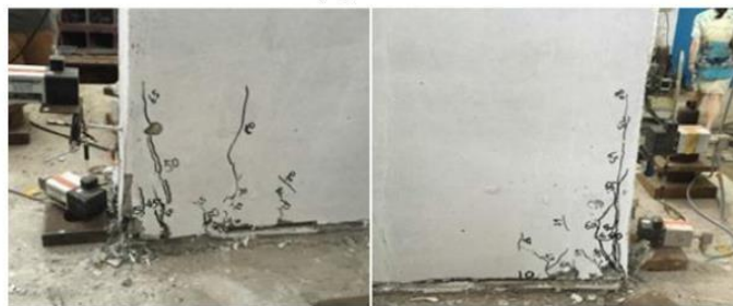
Fig 3. Final damage state of SW2 (Gu et al.2019)
