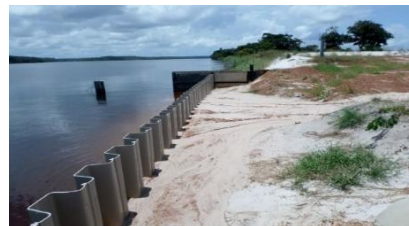
b) River bank protection
