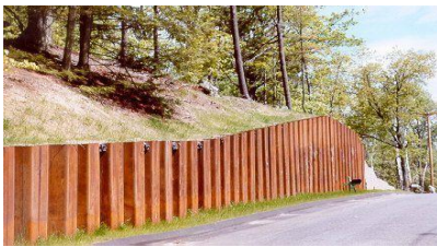
a) Earth retaining wall
