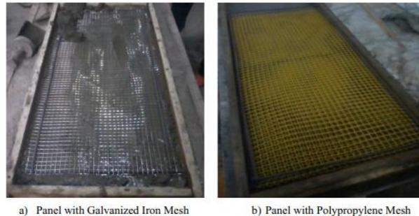
Fig 1: Panels during casting process
