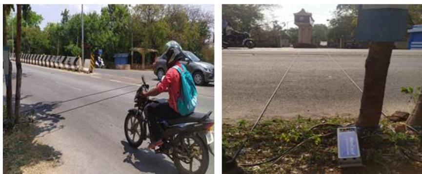
Fig. 2. Installed MetroCount unit for the Traffic study
