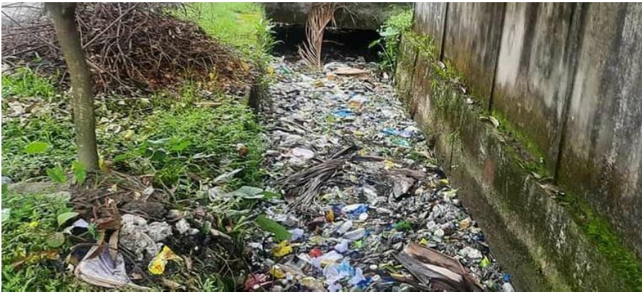
Figure 4. Dumping of solid waste into storm drains
