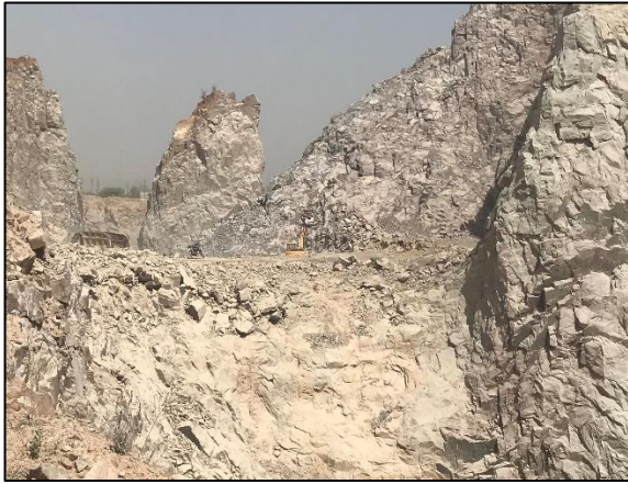
Drilling and blasting
