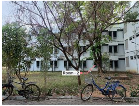
Fig. 6 View of Room 2 from the Northern pathway
