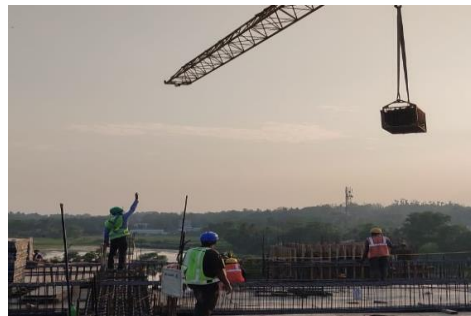
Fig.5 Unsafe behavior of Signal Man by standing on top of bars without safety gears
