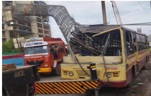
Fig.2 Crane accident at the Metro Rail site on Mount-Poonamallee Road Source: The Hindu,2021)
